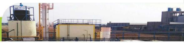
The basic working principle of our H2S Removal System, the Scrubber can be viewed as a caustic type of Hydrogen Sulphide Removal System in which the spent caustic solution is continuously regenerated in a bioreactor.
